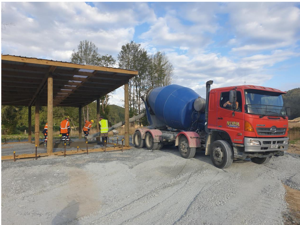
Core Shed construction
