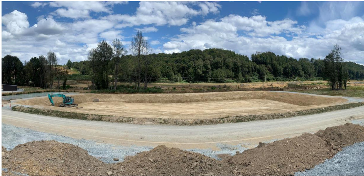
Sediment Pond – Clay liner now completed
