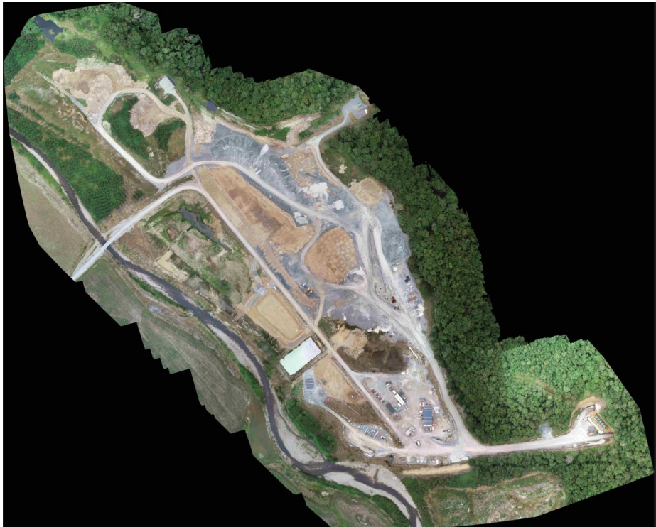
Drone image of site – January 2023
