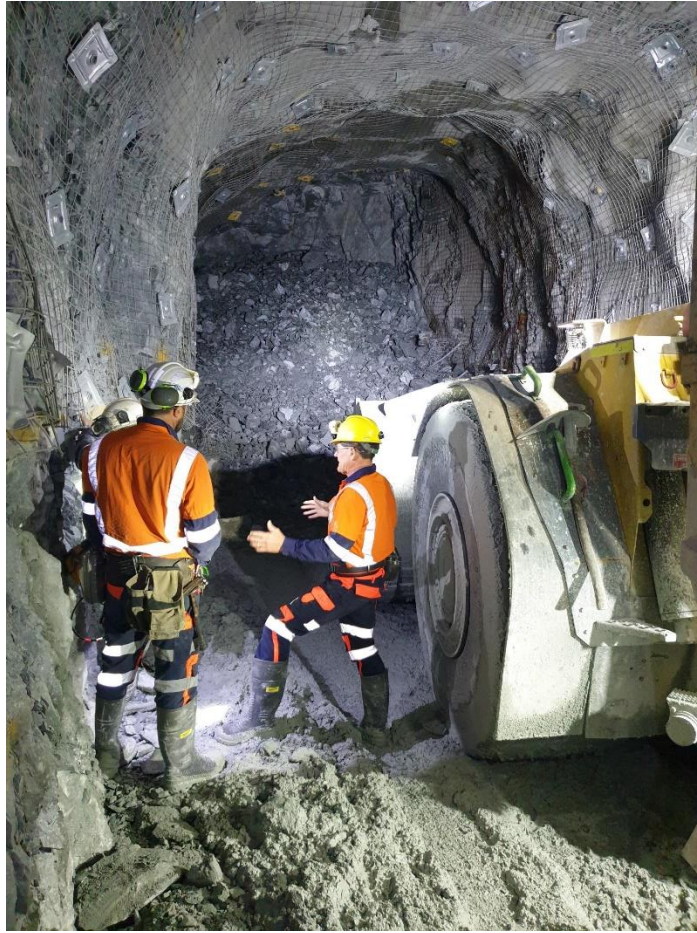
Managing Director, Mark Le Messurier inspecting underground
