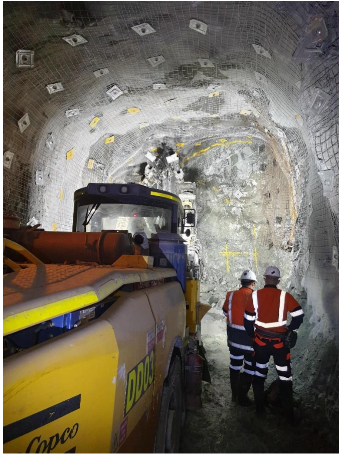
Crews working underground with Epiroc M2D Jumbo
