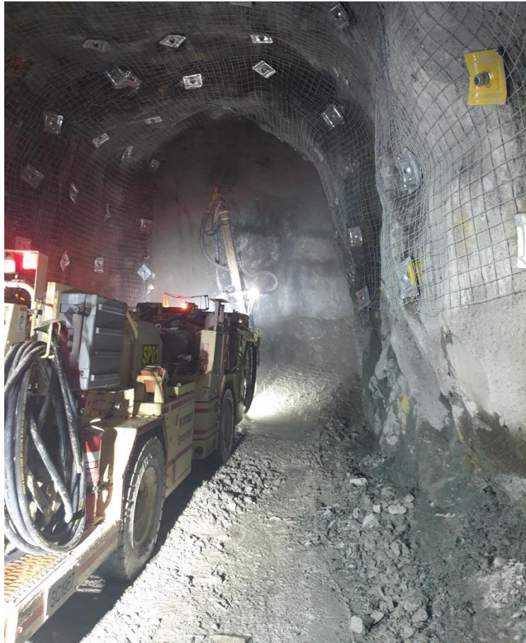
Shotcrete being applied in the North Decline
