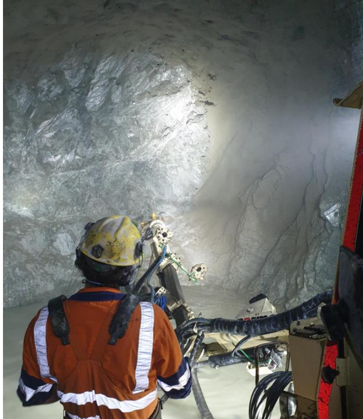
Shotcrete operations in the decline
