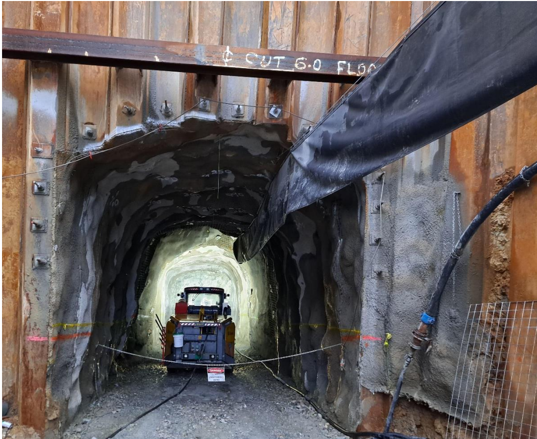
Photo 2 – Epiroc jumbo operating in the Main Tunnel.
